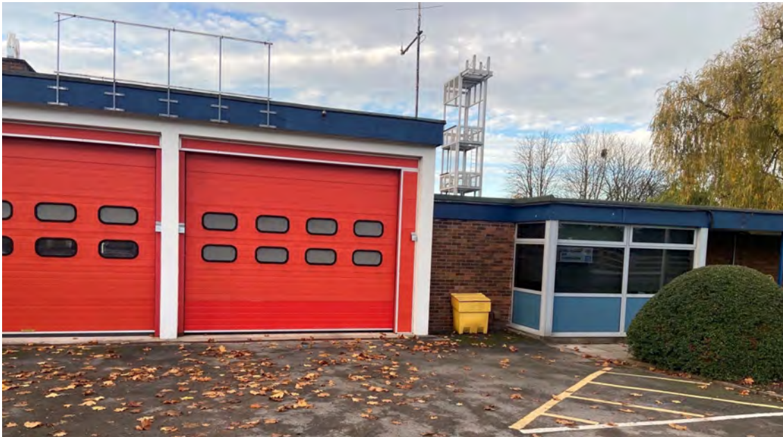
Knutsford Fire Station
