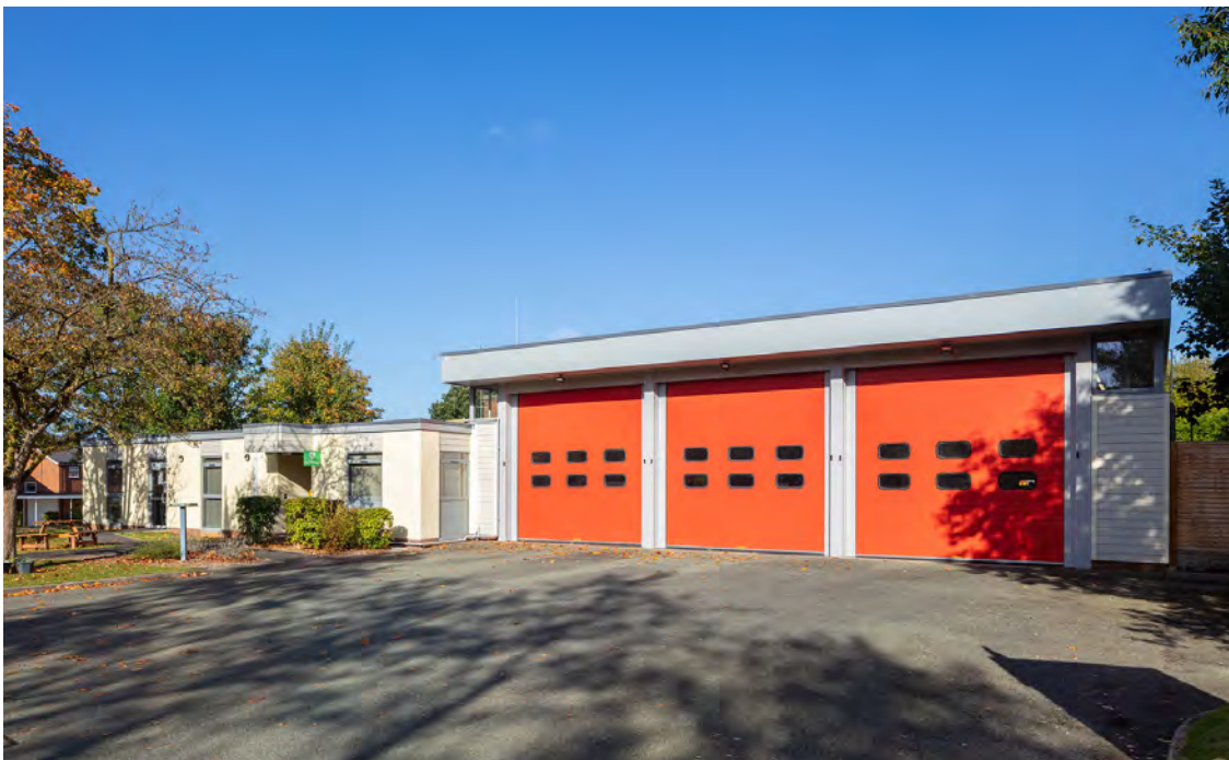
Northwich Fire Station
