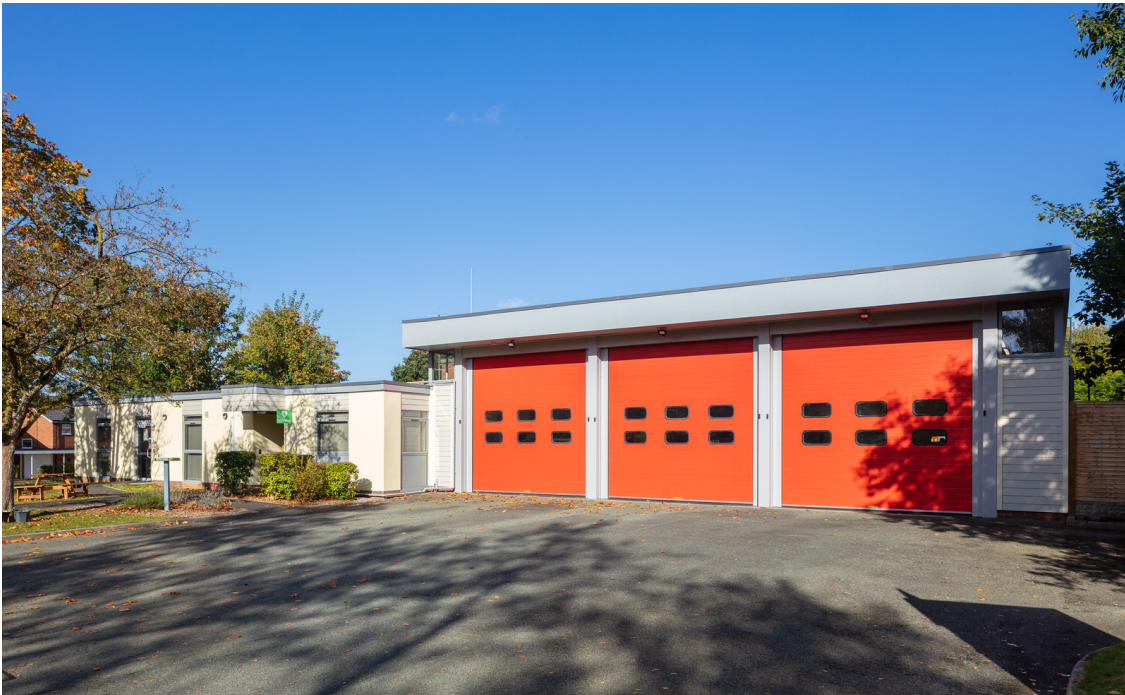
Northwich Fire Station
