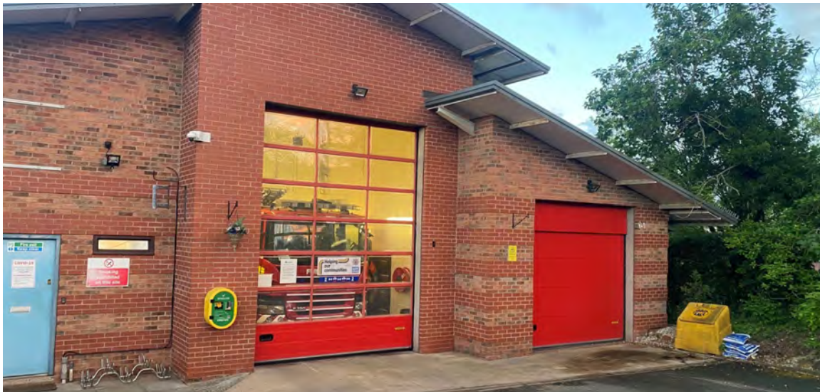
Malpas Fire Station
